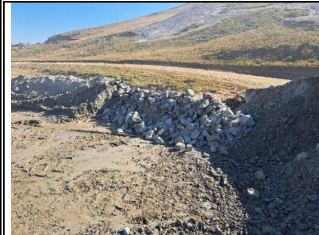
Gabion stone added to berms that acts as sediment trap
