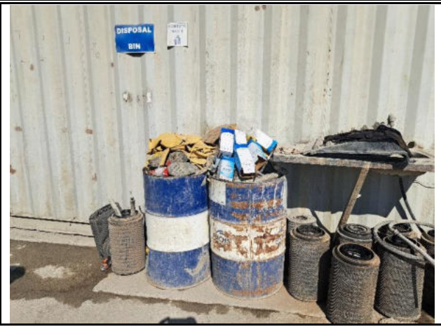
General- and hazardous waste to be kept separate
