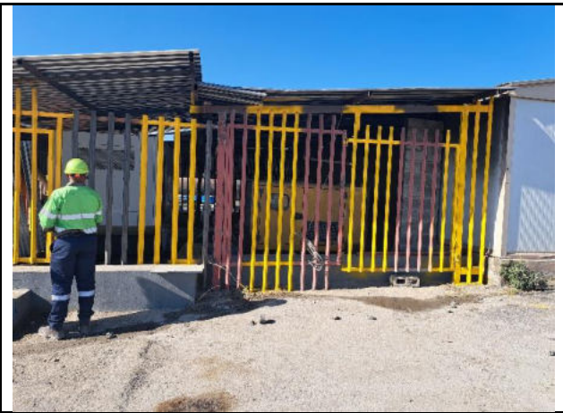
Improvements made to the bund of the generators. The bund must still be cleaned and sealed
