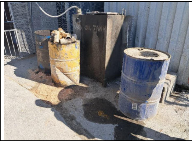
Used oil tank and drums to be placed in a bund
