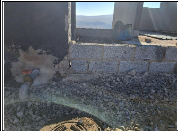
Bund of the used oil storage area to be sealed
