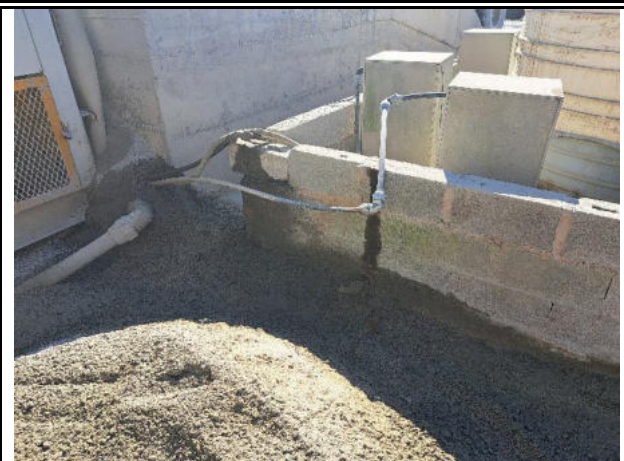
Bunds to be repaired and sealed
