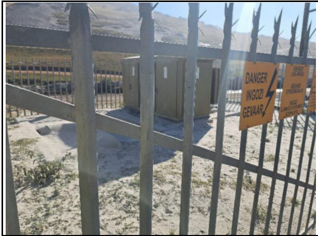
Generators to be fitted with bund walls
