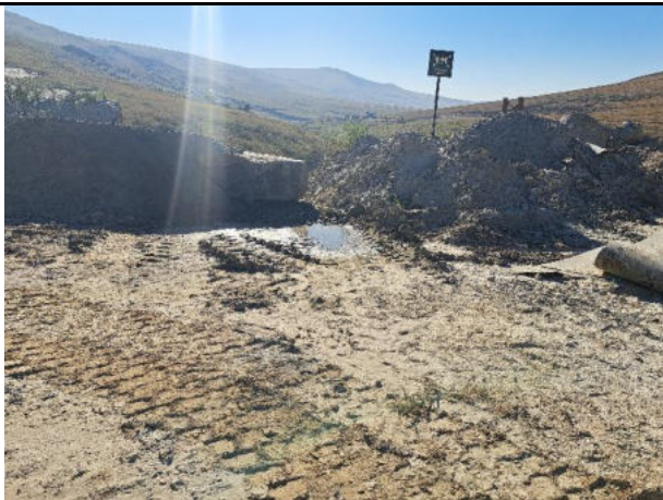
Gabion stone added to berms that acts as sediment trap
