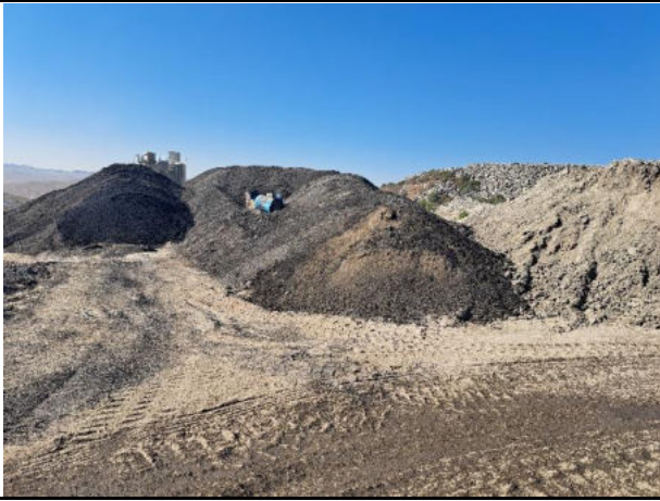
Old bitumen and contaminated soil contained to be reused in asphalt process
