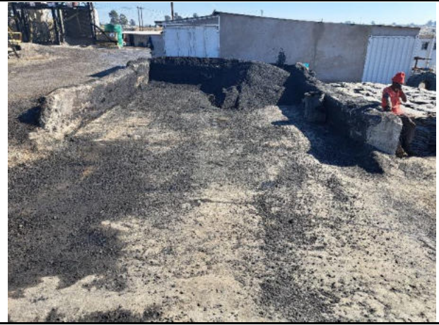
Old bitumen and contaminated soil contained to be reused in asphalt process
