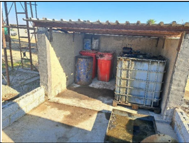
Bund of the used oil storage area to be sealed
