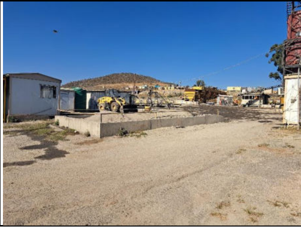
New bund to contain dust material
