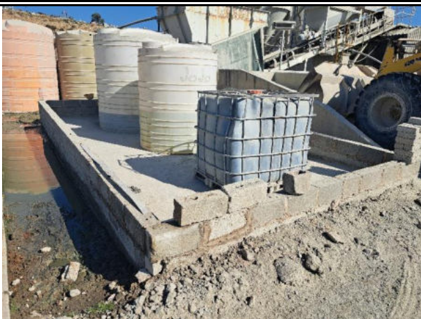
Bunds to be repaired and sealed
