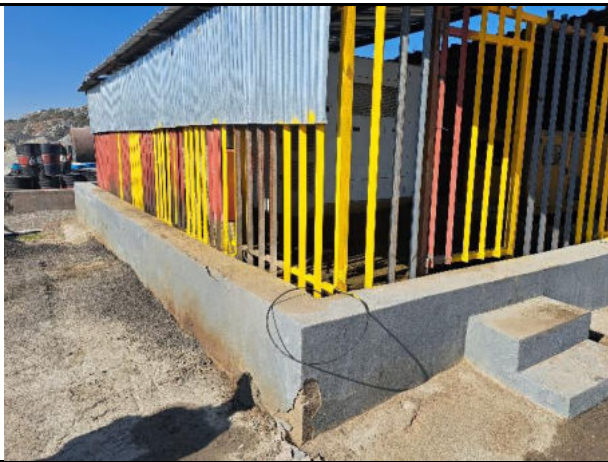
Improvements made to the bund of the generators. The bund must still be cleaned and sealed
