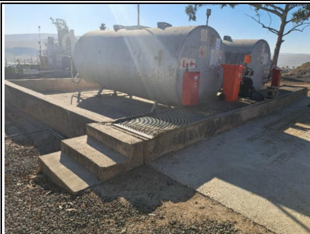
Bund of diesel tanks. Water to be contained and poured into oil sump when needed
