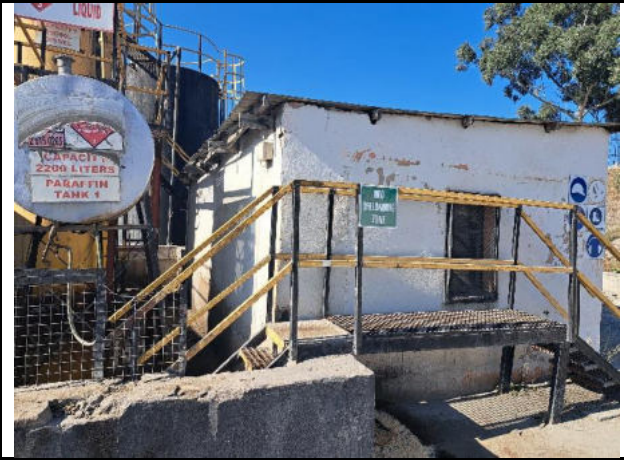
Improvements to bunded area
