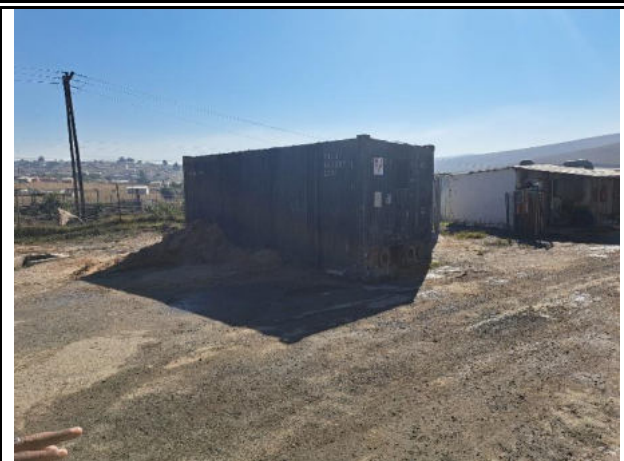
Dust suppression implemented
