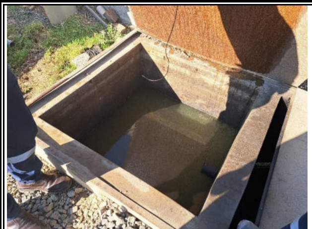
Oil sump. Water from the last chamber to be tested for hydrocarbon traces
