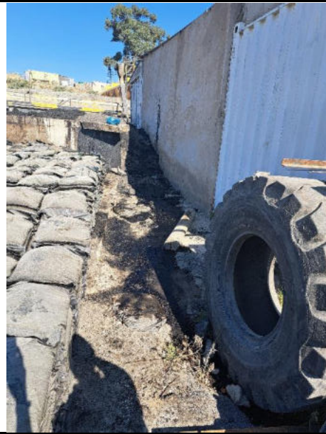
Spills to be cleaned (right picture)
