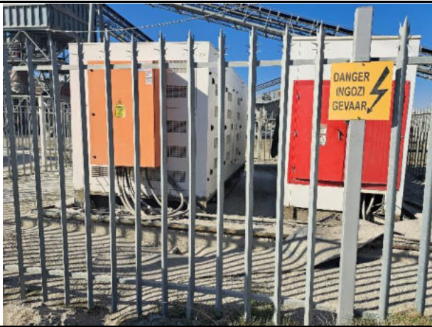
Generators to be fitted with bund walls
