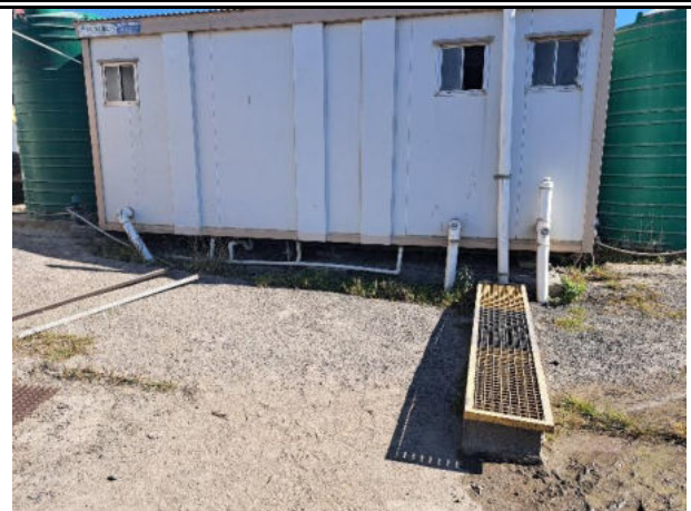
Septic tank cleaned since previous audit
