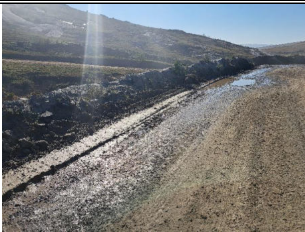
Stormwater berm below the processing plant
