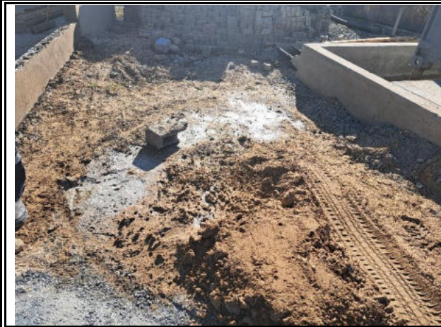
Paint store under construction. No mixing of cement on the bare soil may be allowed
