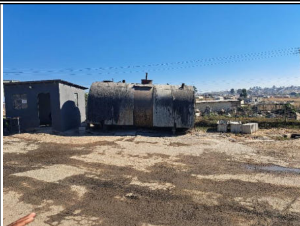
Old tankers being removed from site
