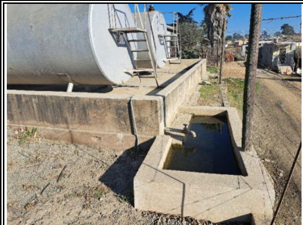
Bund of diesel tanks. Water to be contained and poured into oil sump when needed
